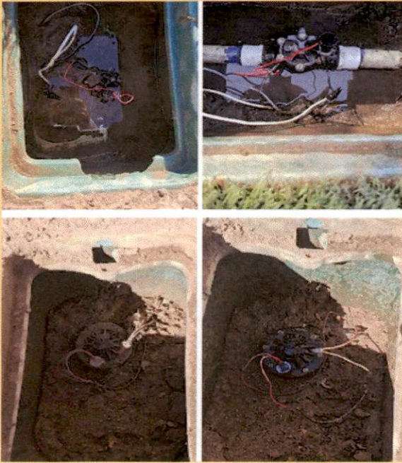
Irrigation repairs were done throughout the city basin.
