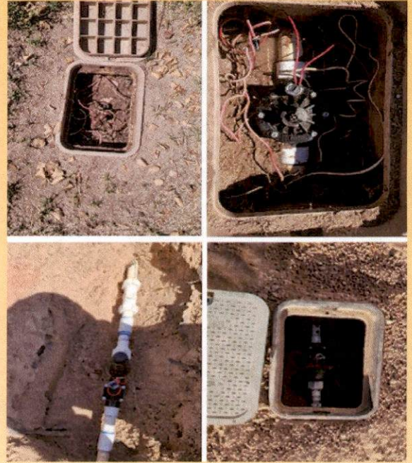
Irrigation repairs were done throughout the city basin.
