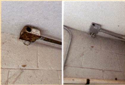
Repaired electrical box and pipe at the bool filter room.
