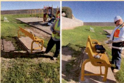
Installed new benches at parks/retention basins throughout the city.
