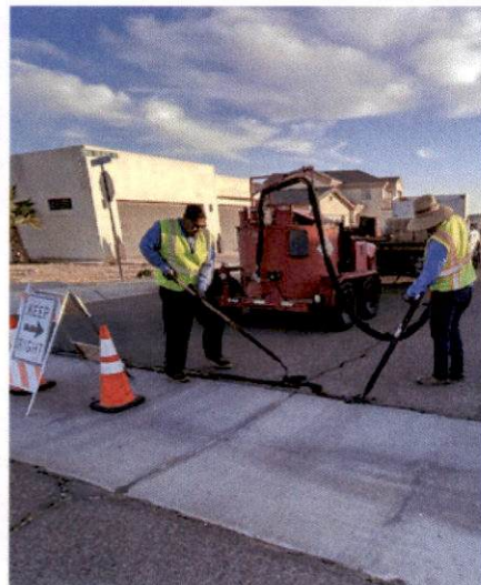
Crack Seal
